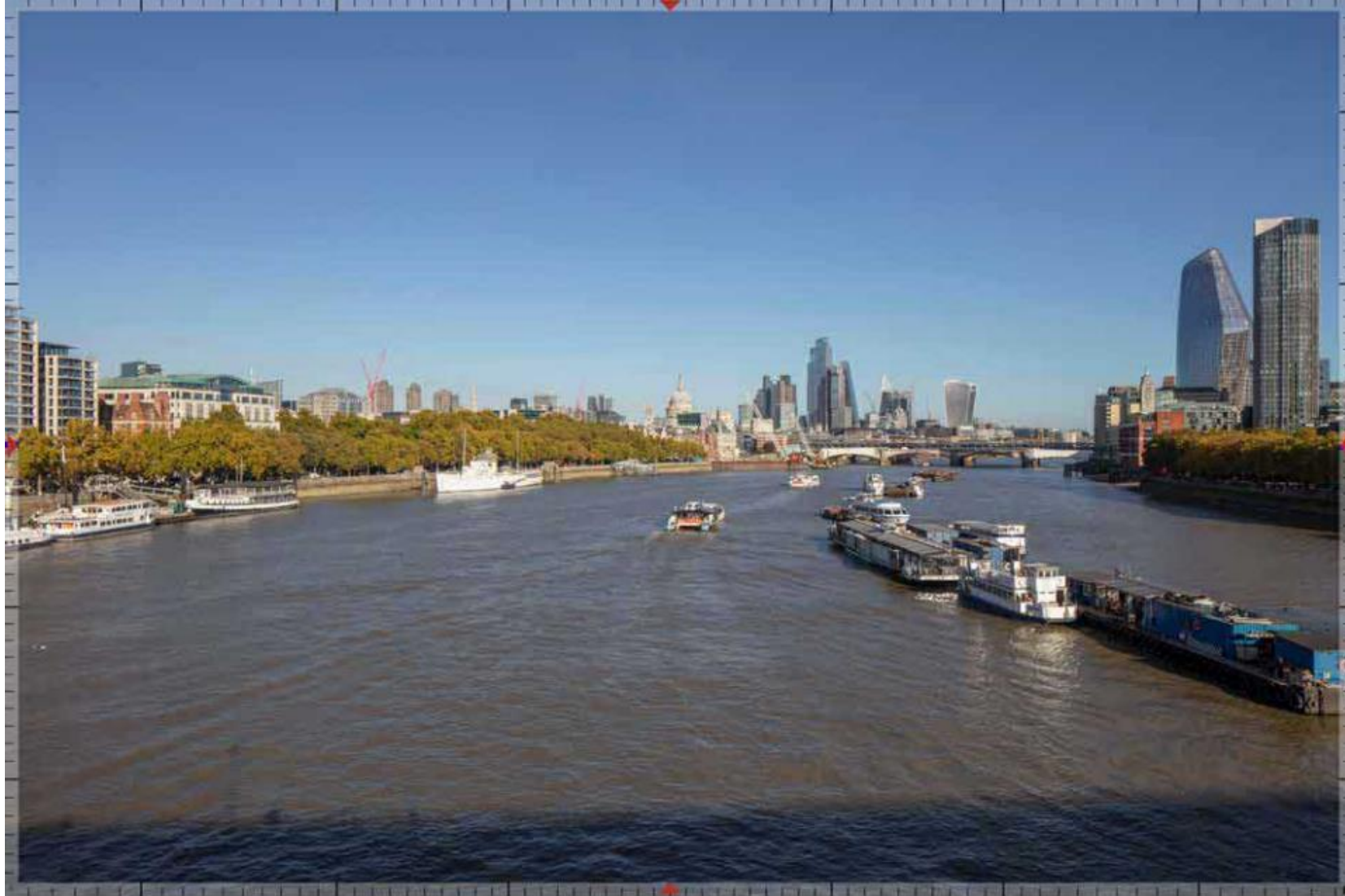
Existing: LVMF 15B.2 – Waterloo Bridge: downstream – at the centre of the bridge
