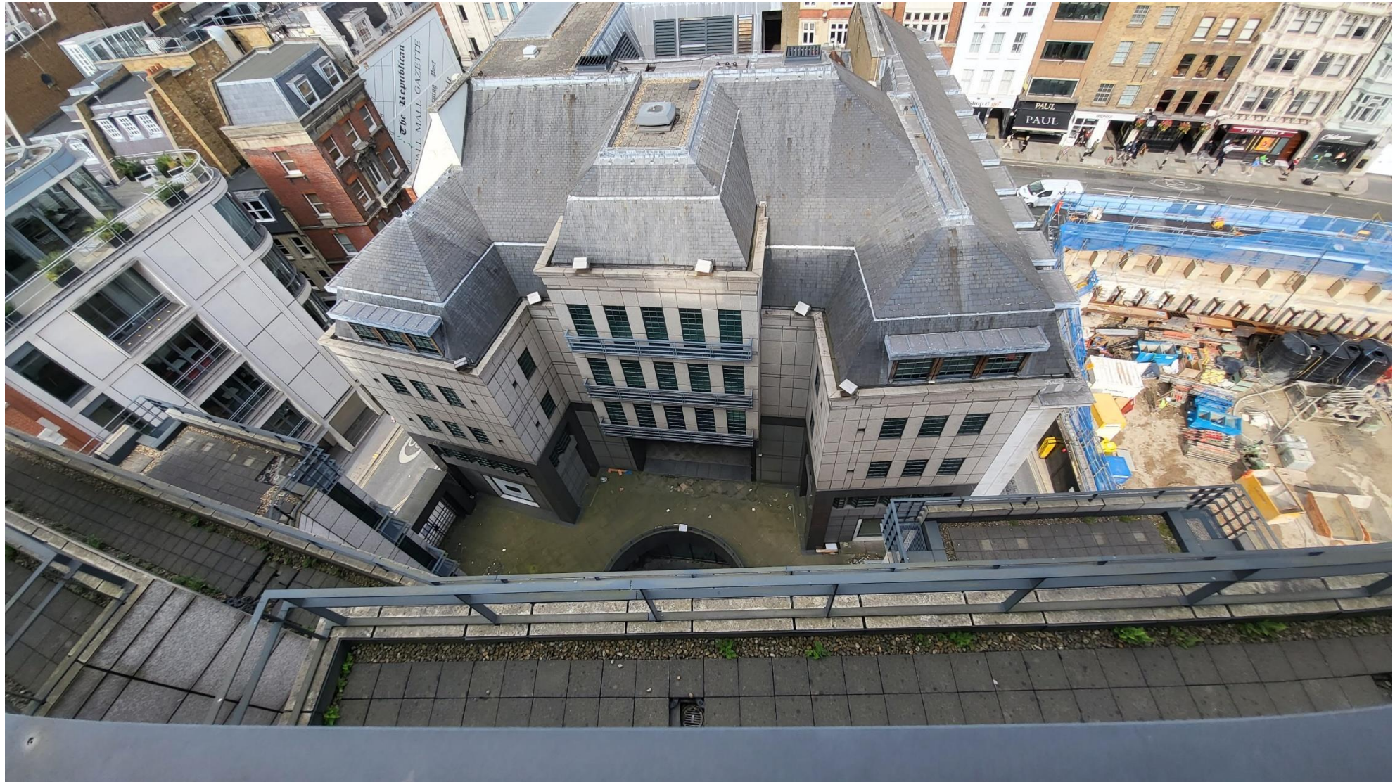
View to the internal courtyard and rear elevation of north block
