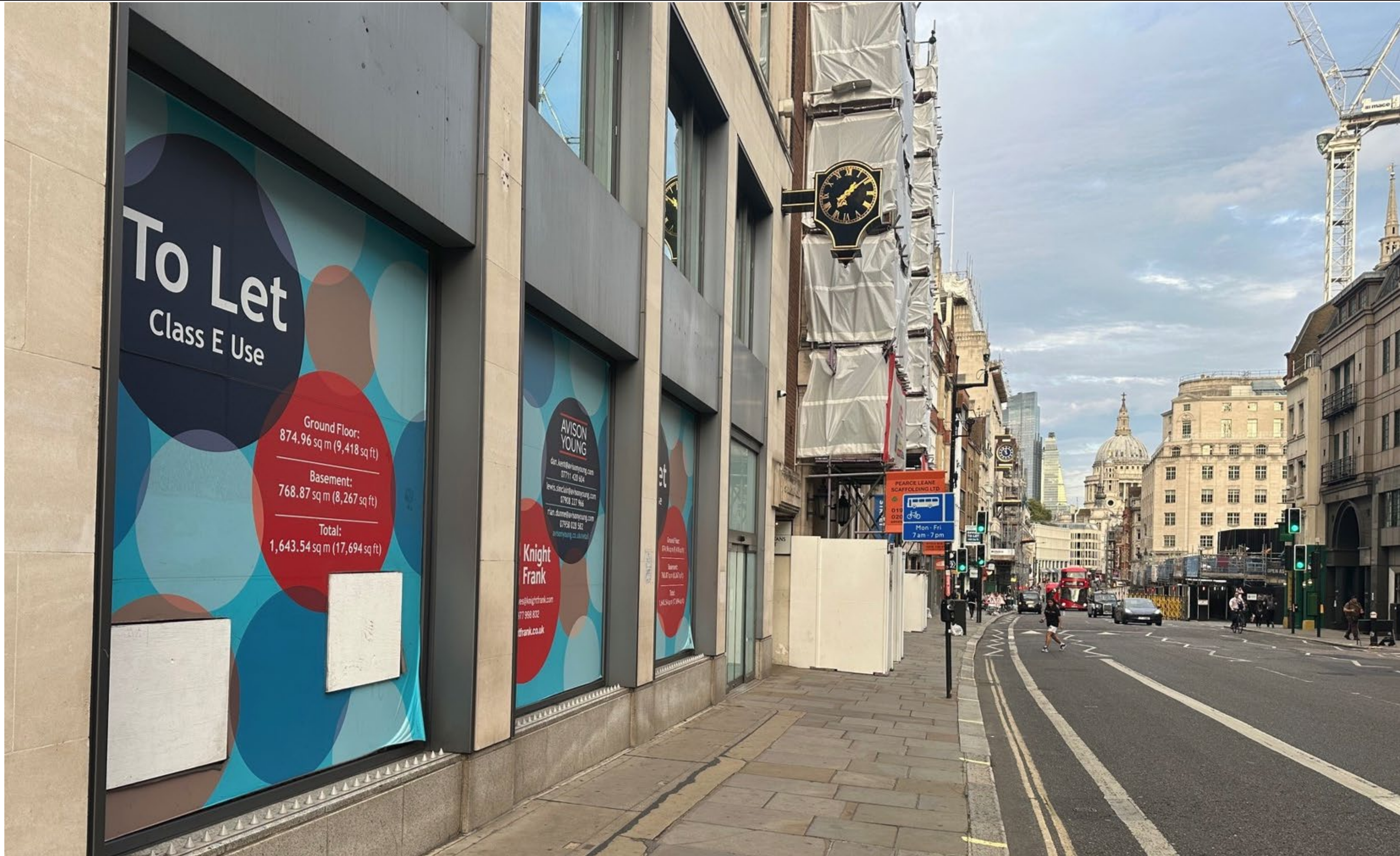
Existing Unit – Fleet Street View East
