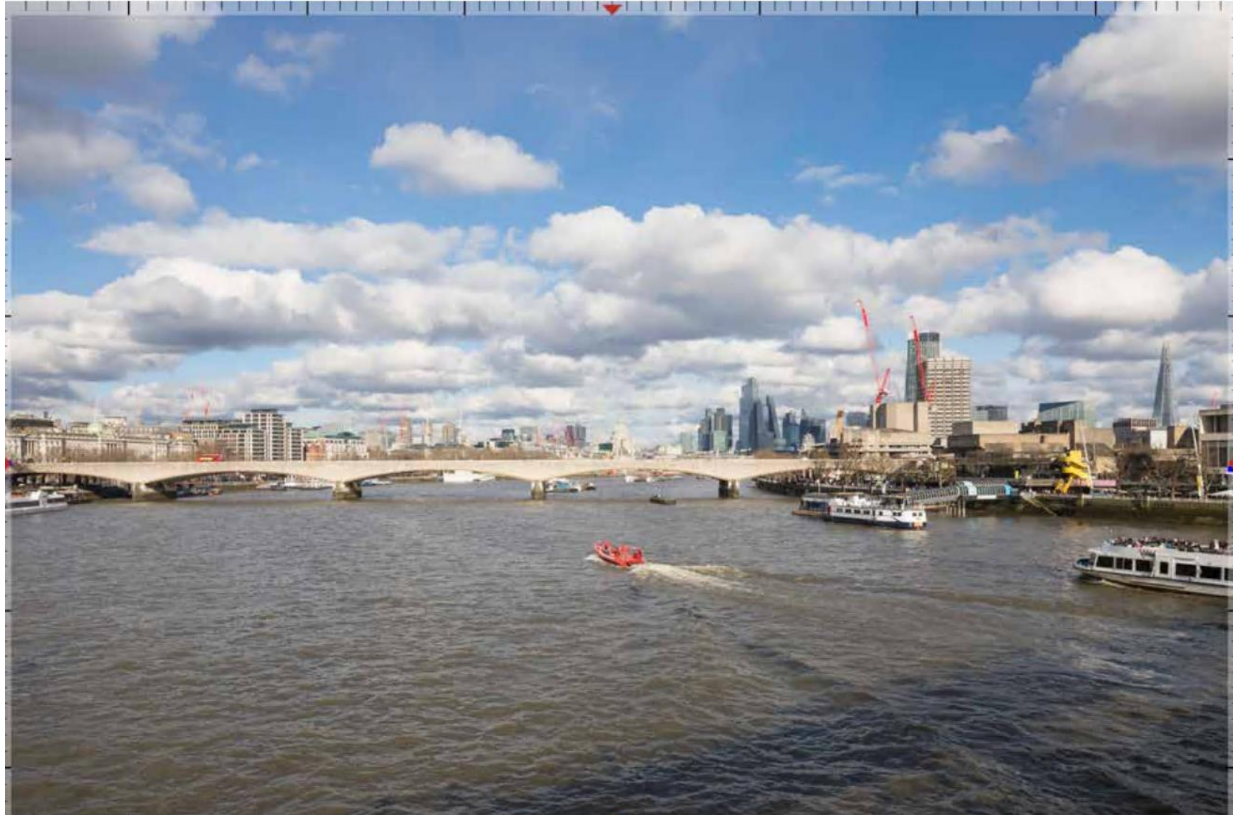
Existing: 17B.2 Golden Jubilee/Hungerford Footbridges
