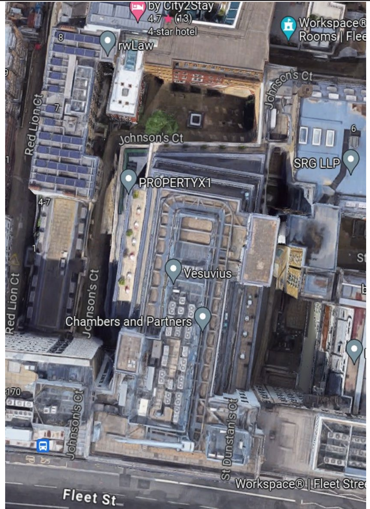
Existing Building – aerial view
