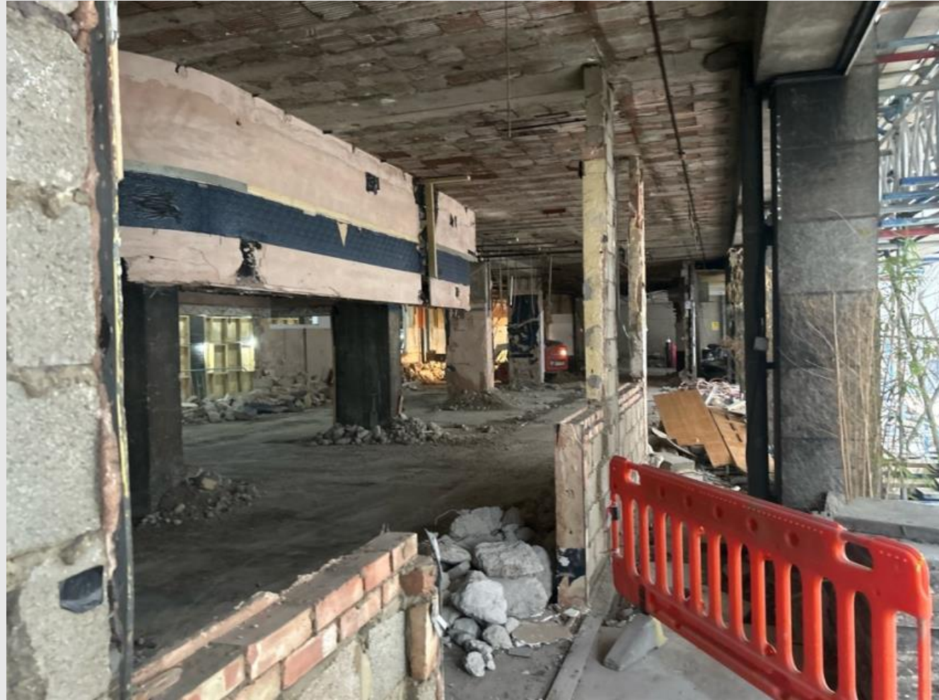
IMAGE TEN: Interior view of Ground Floor (02/10/2024)
