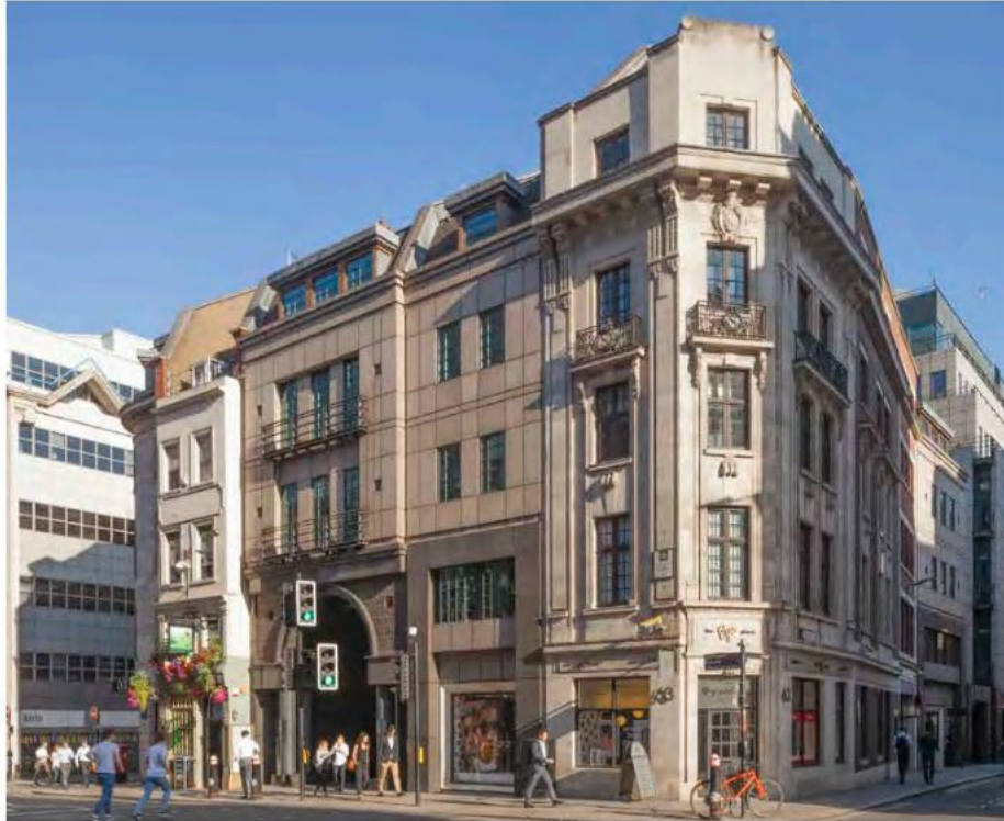
Existing Fleet Street View
