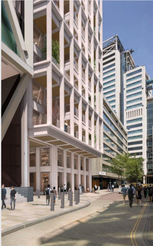
IMAGE FOUR: View from Moorfields looking northwest
